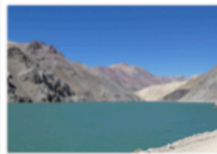
La Laguna Dam
