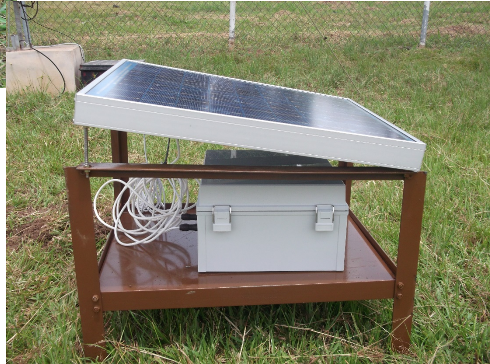
Power source and data logger
